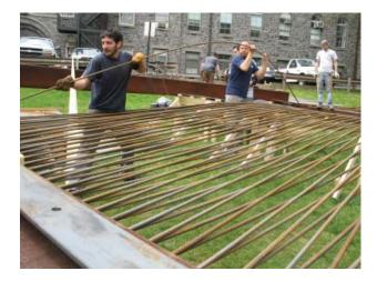
Figure 8. Help from friends and students from Buffalo to thread rebar into the perimeter steal beams
