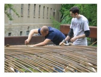
Figure 7. Lehigh students preparing rebar for welding during installation
